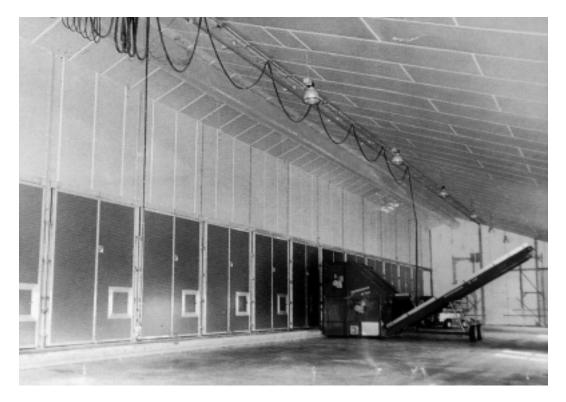
Exit air is treated in a compost biofilter, and temperature and oxygen content of the air are monitored.
